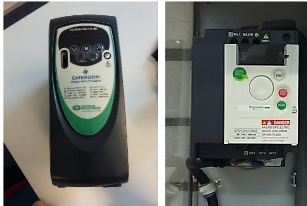
Figure 5-16: On the left, the original frequency meter that was burned out. On the right, the installed frequency meter.
