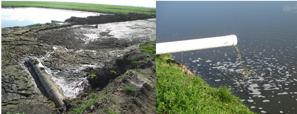
Figure 14. WSPs used for wastewater treatment from dairy farms. Pictures taken in a conference about dairy farm effluent treatment in 2014. Left: anaerobic silted pond. Right: Discharge of the treated effluent in a water body.
