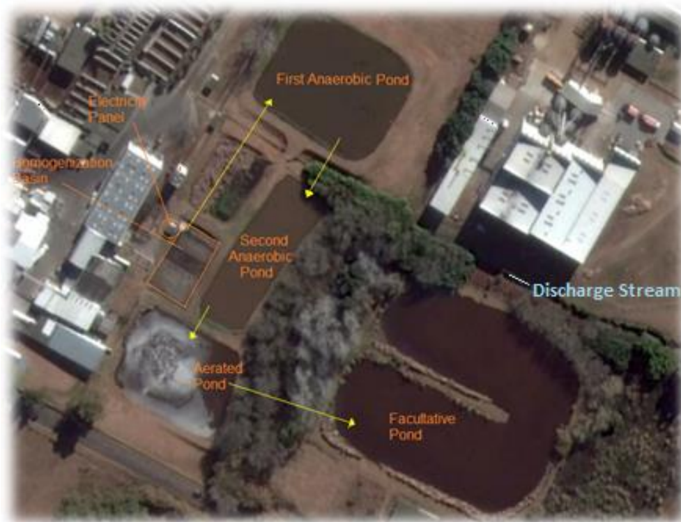
Figure 7: Ponds treatment system for Schneck slaughterhouse
