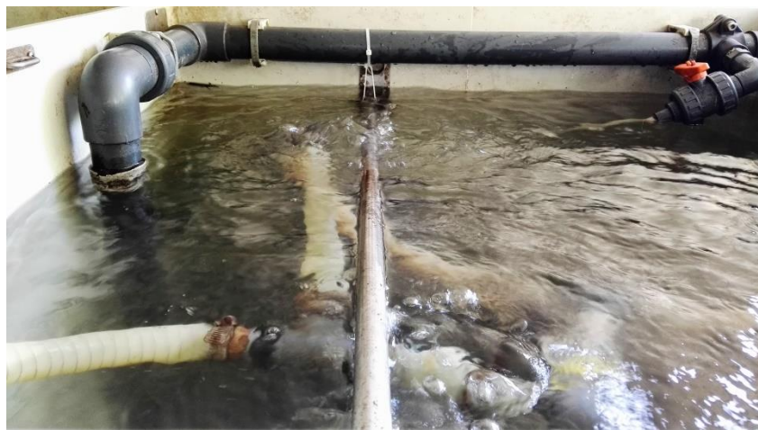
Figure 14 Hydraulic tests with clear water.
