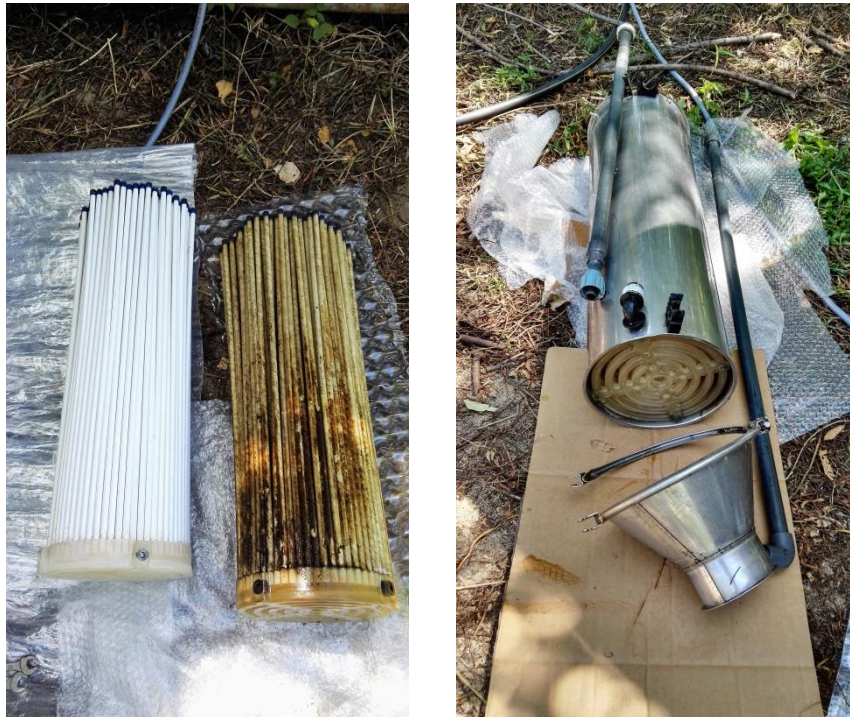
Figure 13 Replacement of the old membranes.
