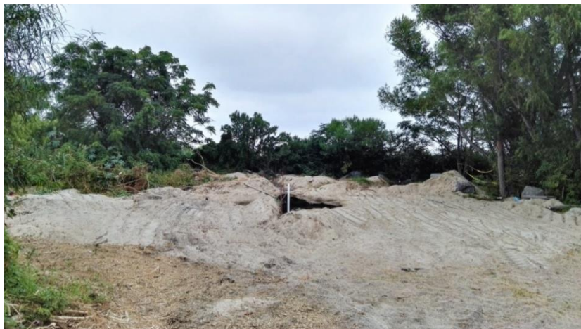
Figure 10 Effluent infiltration area being under maintenance.
