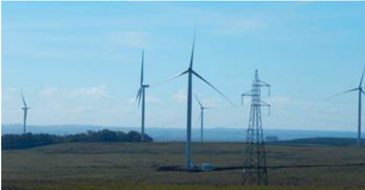
Figure 4—6 Pampa wind farm
