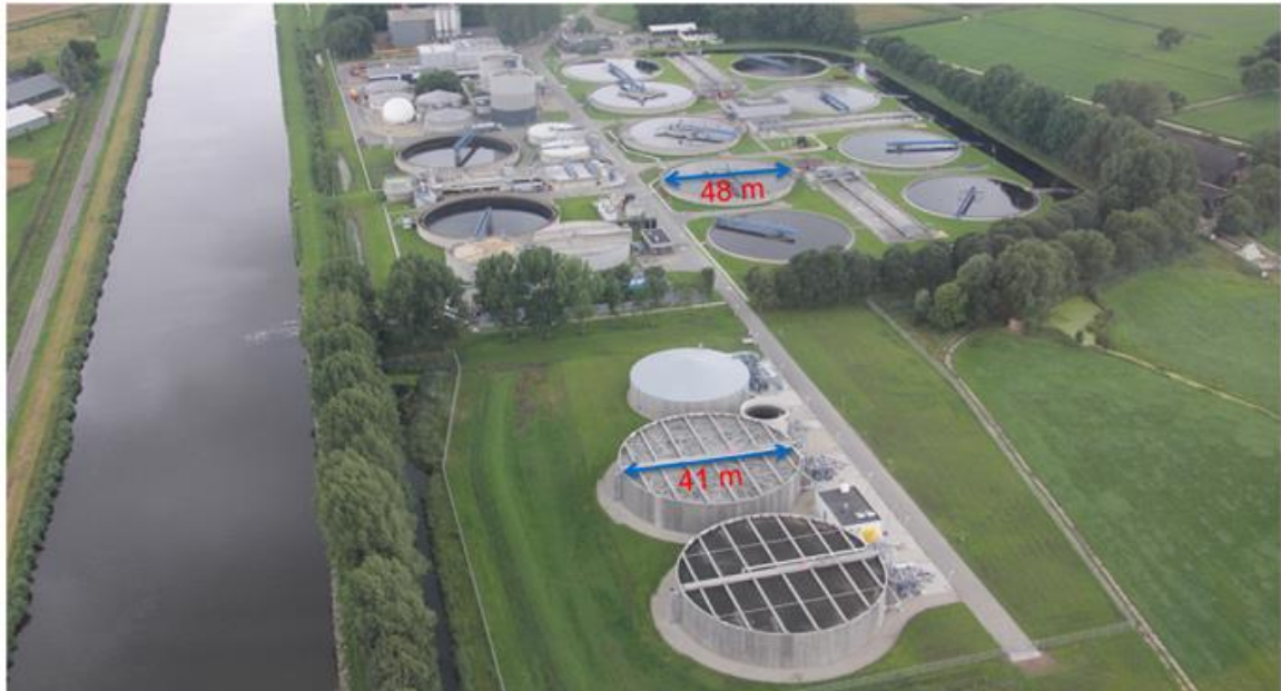
Figure 2-2: Aerial view of Garmerwolde WWTP. AGS plant is located in the front (Pronk, et al., 2015)
