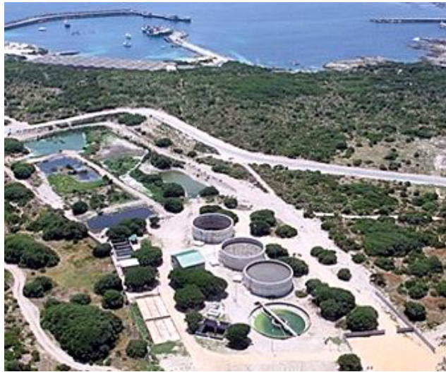
Figure 2-1: Aerial view of Gansbaai WWTP (Dutch water sector, 2015)
