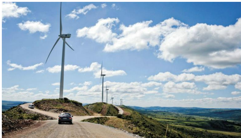
Figure 3- Example of Horizontal Axis Wind Turbines (HAWT) located in Maldonado, Uruguay [6].
