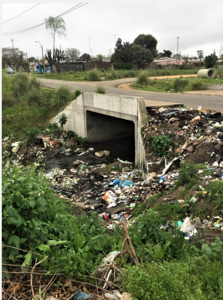
Figure 2.13: Road and sanitation work in Montes Pareja Street and Iyuí Stream. Date: September 2021
