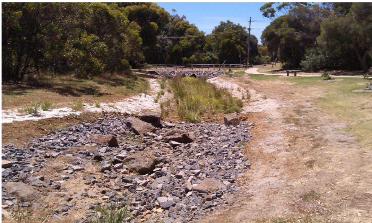
Figure 0.4.10: Jan Juc Creek Daylighting Project
