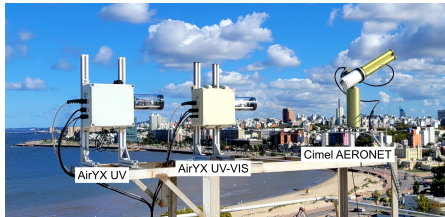
Figure 2. Instruments are installed on the roof of the Faculty of Engineering building located in Montevideo, Uruguay (34.9175° S, 56.1669° W). AirYX equipments are Multi-Axis Differential Optical Absorption Spectroscopy (MAX-DOAS).
