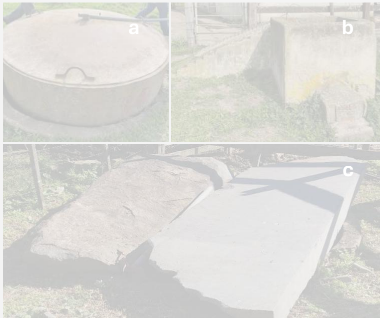
Indian type digesters. a: Floating biogas-holder in Escuela Agraria de Durazno (2024). b: Elevated mixing tank in Escuela Agraria de Durazno (2024). c: Unoperated reactor in Colonia dairy farm (2019).
