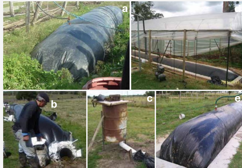
Low-cost tubular digesters. a: First Uruguayan tubular digester in López's dairy farm, Castillos (2006). b: Manual feeding. c: Inlet mixing tank in Azzanelli's dairy farm, San Ramón (2008). d: Concrete pit for tubular digesters in González's dairy farm, Castillos (2010). e: Greenhouse for digester insulation in Parque UTE, Lavalleja (2010).
